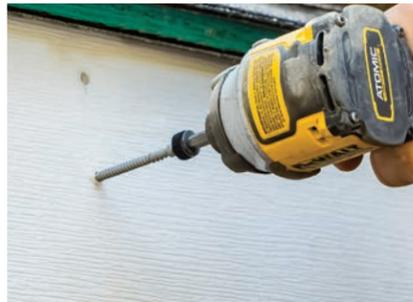
Drive fastener at 90° angle to preset level below trim surface.
