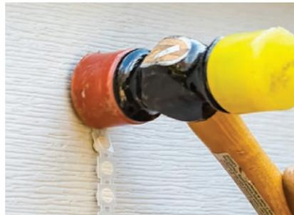
Place plug with trim surface side-up into hole. Gently tap plug until flush with the trim.
