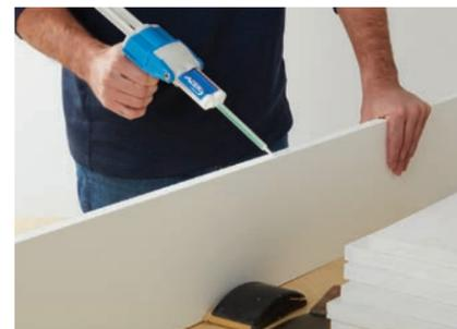
Use AZEK Fast Cure and Slow Cure to fill gaps and other trim connections that do not require tight compression. Use a putty knife to distribute and sand when dry for a smooth finish.
